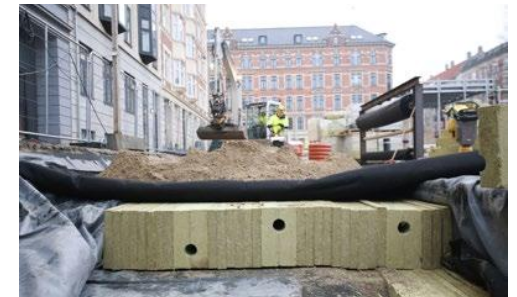
The photo underneath shows how Rockflow has been installed under the surface of the square. Unlike insulation, the stone wool in the Rockflow system is specially engineered to absorb and retain water. A system of pipes and gullies bring the storm water to the stone wool buffer where it is absorbed quickly and released slowly, either to the sewer or surrounding soil.
